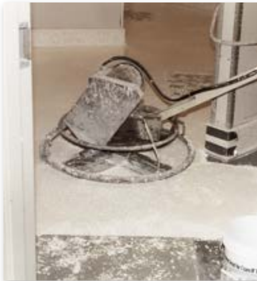
Queens Hospital Center - April 2004 Terrazzo is hardened with the "helicopter".
